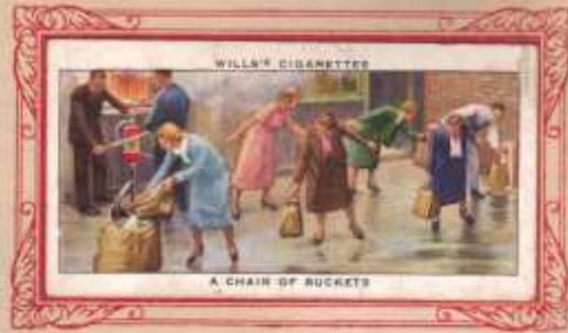
**A CHAIN OF BUCKETS.** When using a hand pump, it is necessary to have a ready supply of water which can be contained in any convenient receptacle. In the illustration, a small canvas dam is being used and kept full by a chain of persons passing filled buckets from hand to hand, others returning the empty buckets to the source of supply. The illustration shows a small hand pump in use; water is being taken from the canvas dam and a jet of hose led into a building on fire. (No. 20)
