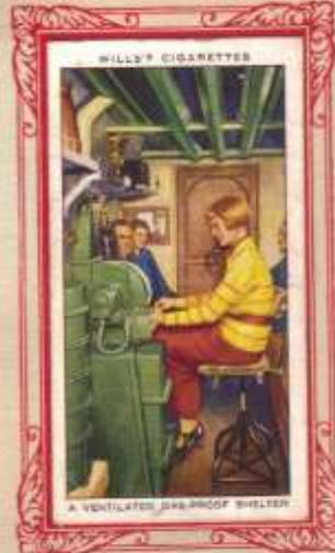
**A VENTILATED GAS-PROOF SHELTER.** The illustration shows a gas-proof shelter which is ventilated by air drawn in through a gas filter so that it is delivered inside the shelter for the occupants to breathe, free from poisonous gas. The filtration plant is normally driven by electric power, but if this should fail, filtered air can be drawn in by manual labour, worked on the same principle as in a sewing machine or a bicycle. The picture shows the latter method in operation. (No. 11)
